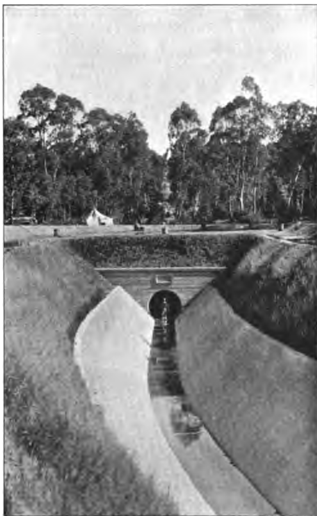
INTAKE CHANNEL, BAROSSA DAM.
